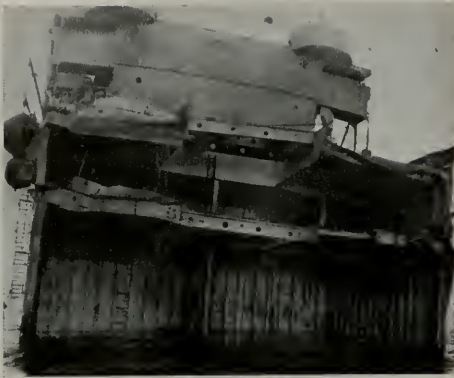
Aft section of Valery Chkalov showing break in end of No. 3 hatch.
